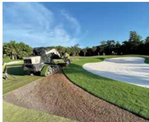
Top: As a part of the bunker portion of the renovations at Olde Florida, crews removed sand from the bunkers, and that sand was later used to modify soil in historically wet areas around the golf course. Photo courtesy of EPIC Creative
